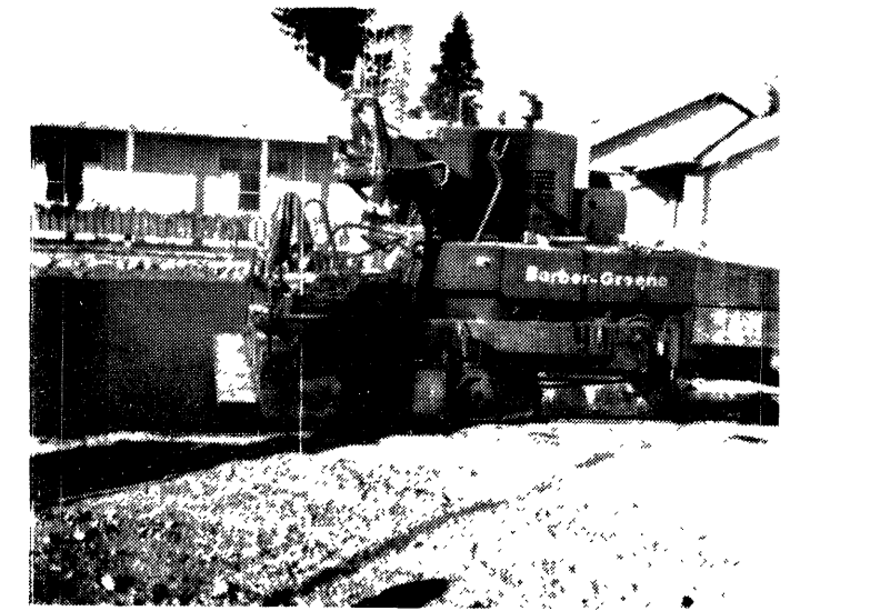
INTERSTATE ASPHALT COMPANY of Aberdeen is surfacing the intersections and alleys in Forks this week. According to a spokesman for the company this is about the fifteenth year they have worked in Forks.
